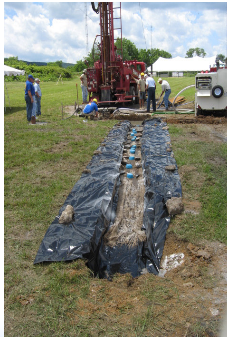
Above: Settling pit is dug out to allow larger sediments reaching the surface to settle out before the water is channeled into the mixing ditch.
