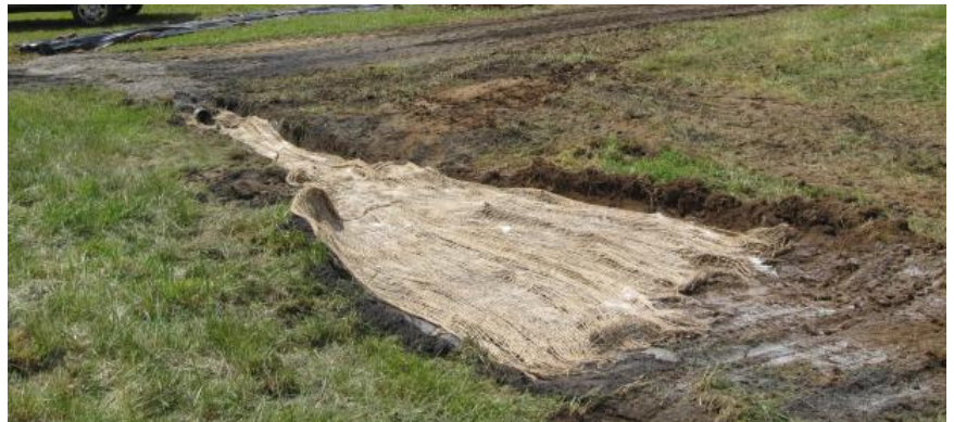
Above: Photo One - End of mixing ditch channeling into pipe, leading to dispersion field. Photo Two - Jute lined dispersion field which captures reacted sediment.
